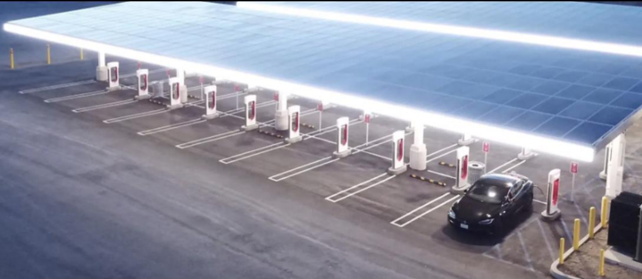
Existing Tesla Solar Canopy Charging Stations
