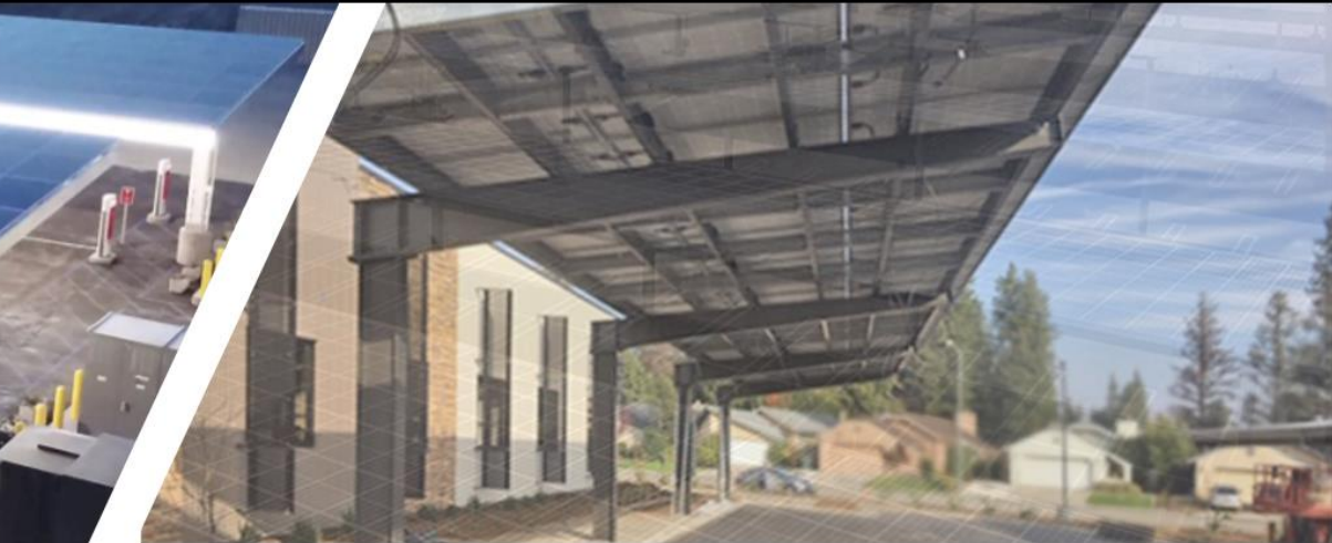
Solar and EV Charging for Commercial real estate and municipal applications.
